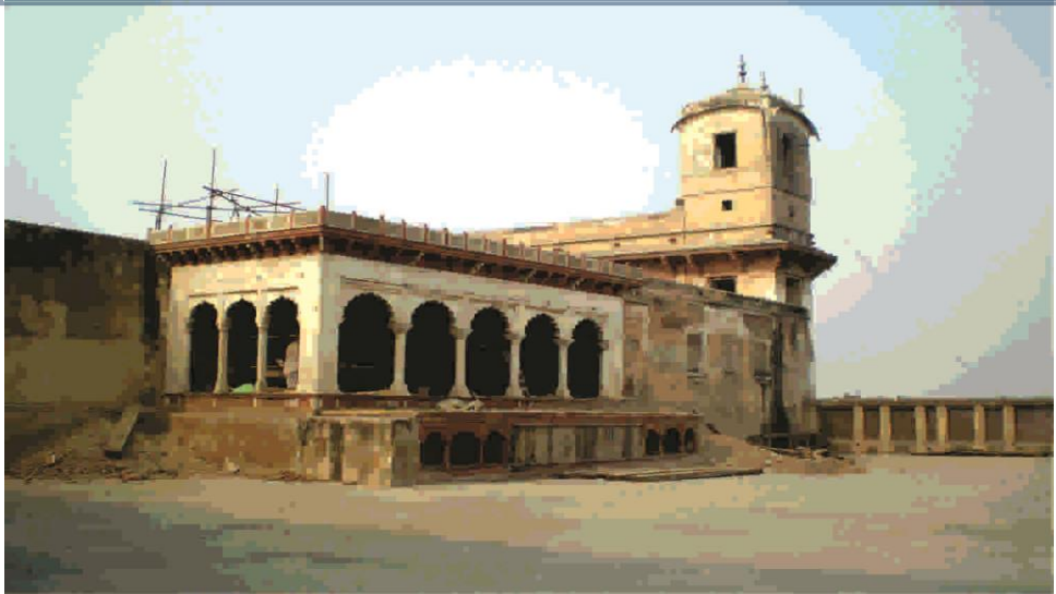
Sikh period Athdara & Pavilion above Shish Mahal also added during Sikh periodalso added during Sikh period
